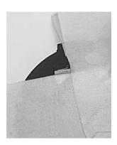
Re-apply a couple of layers of masking tape to protect the adjoining surfaces.
